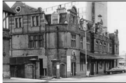
Market Place Station Frontage
