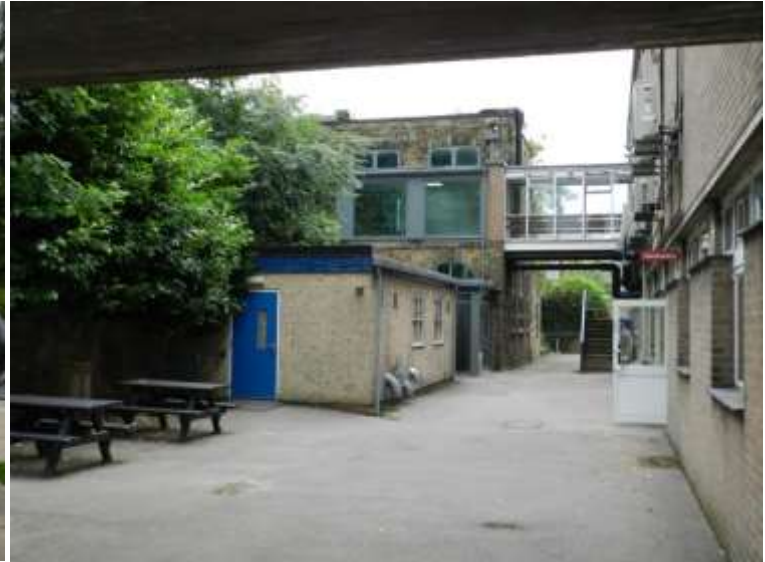
Looking to the North Wing from the top of the Bank
